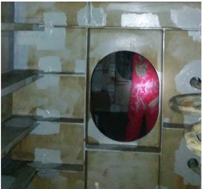
Work "to" and "after" in the ballast tank of the tanker
